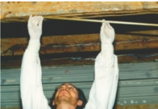
Structural reinforcement (courtesy Rotofix UK and Topglass SpA)
