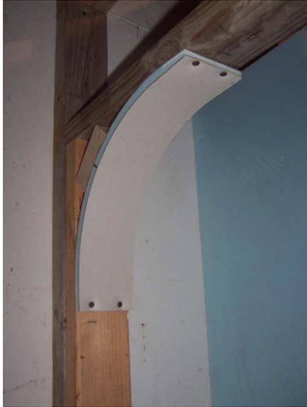
Fasten corners in place with drywall screws
