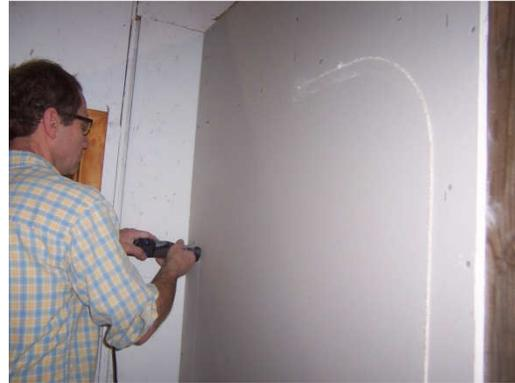
Install face-sheet, roto-zip opening. Screw into blocking
