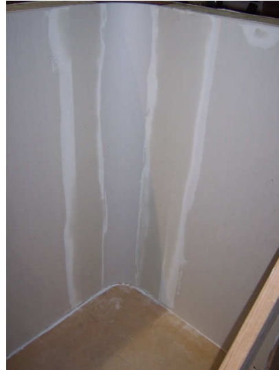
Tape & Mud like drywall
