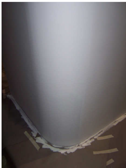
Finish & Prime like drywall
